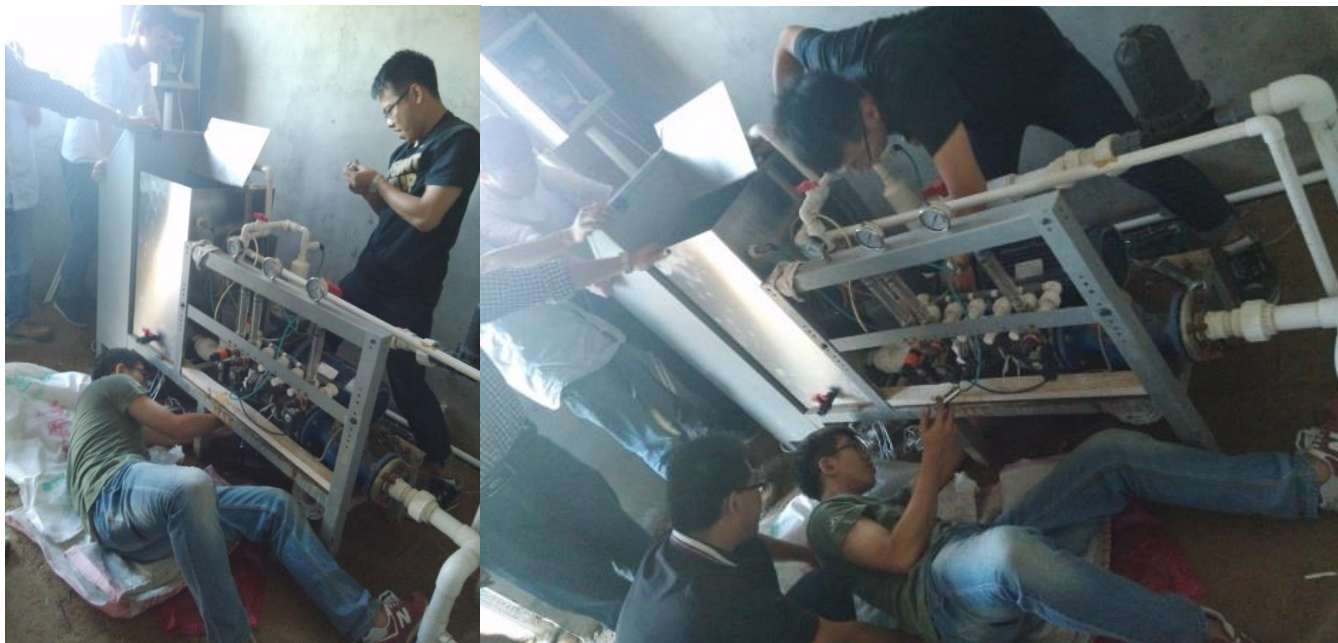
Students installing the MACQU system.
