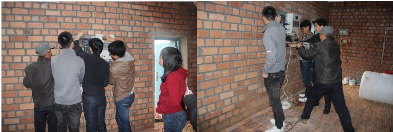
Students are installing the MACQU system.
