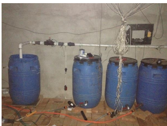
The fertilizer and acid tanks
